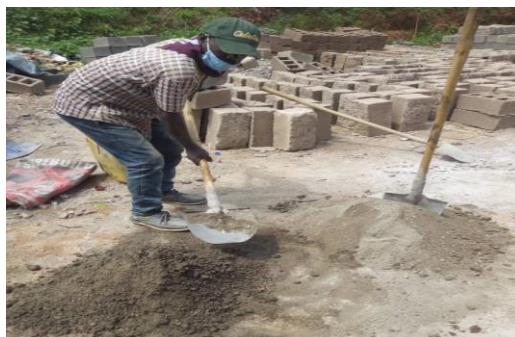
Figure 4. Cement blocks manufacturing at Gisozi site
